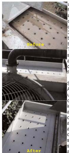
used Cortec's high performance, moisture cure urethane coating - VpCl-396 - on the distribution deck of the cooling tower. The pictures shown are before, and then after, one year of performance.
